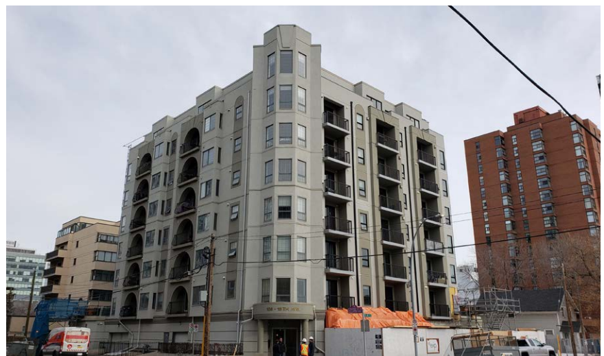
Image 6: Partial but holistic approach to building envelope retrofit updating the architectural style and improving the user experience by increasing daylight through the balconies.
