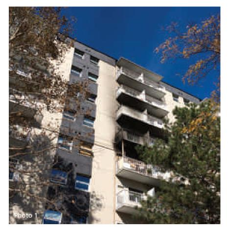
Many older condominiums in Canada have also been keen to improve the exterior appearance of their buildings and improve energy efficiency. In the 1980s and 90s, many older apartment buildings were overclad with non-combustible fibreglass batt insulation behind industriallooking steel siding. More recently, condos have been over-clad with EIFS (Exterior Insulating Finish System)
