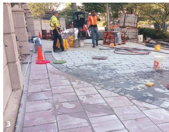
Clockwise from left: 1) Concrete with GFRP Reinforcing; 2) Adhesive installation; 3) Grouting the joints. 4) The finished driveway. Photos: Supplied.
